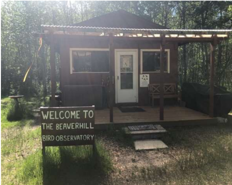
Above: The humble shack that was the old BBO lab building until fall 2020.
