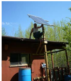
Al installing solar panels
