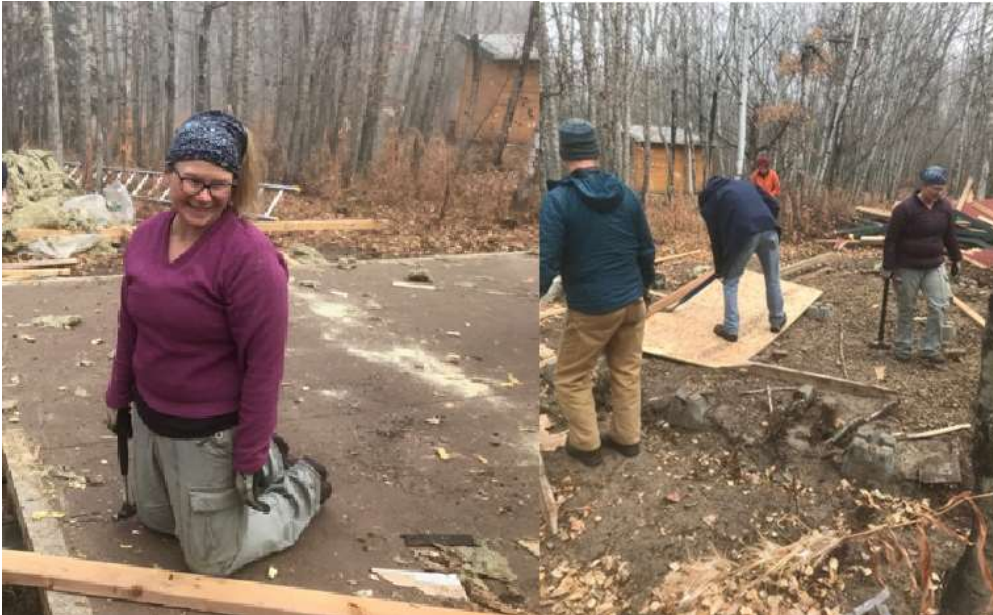
Board members and volunteers demolish the old Nuthatch Nest bunkhouse.
